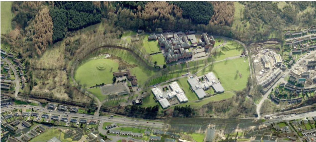
Aerial view from the north. The site is to the left of the picture within the "L" shape former by Inverkip Road and Pennyfern Road
